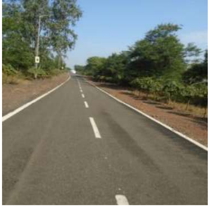
Guest House to Main Gate
