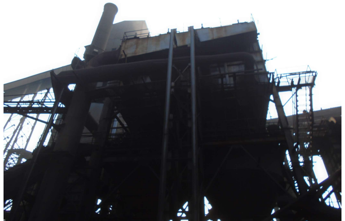
(fig. 8: DRI New Bagfilters - Cap:85,000m 3 /hr)
