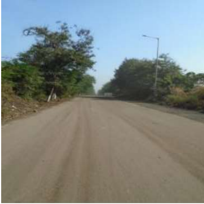
Way to Power Plant
