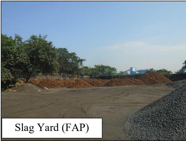
Figure 3: (Solid Waste Yard)
